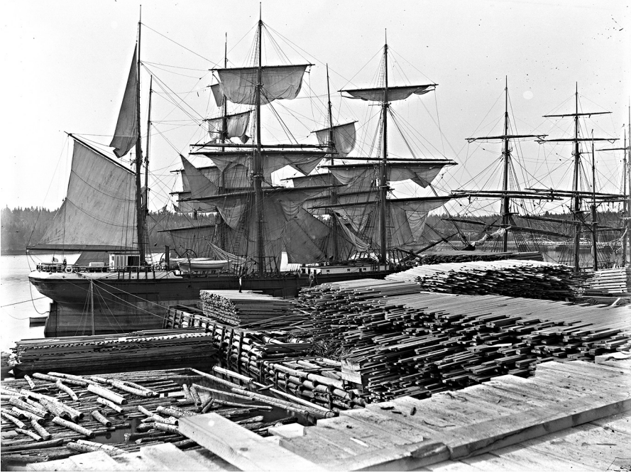
Barques loading deals at (Edward) Sinclair Lumber Co. sawmill, Northwest Bridge, Newcastle. PANB Ole Larsen Fonds: P6-211.
